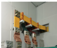
变压器减震 Transformer vibration damping
