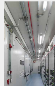
Interior Design: ➢ Rock wool board walls and ceiling + exposed pipelines
