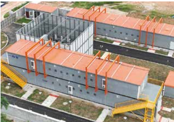
✔ Data Center Industry
