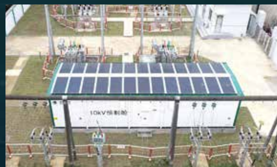
Substation technical renovation
