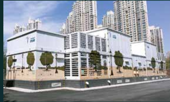
New construction of substation
