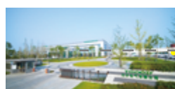
Sichuan Chengdu Manufacturing Factory
