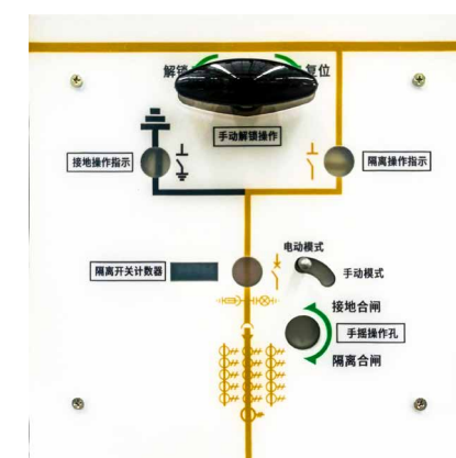
Earthing Switch CLOSED and Circuit Breaker CLOSED
