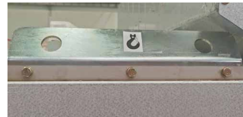
View of Switchgear Lifting
