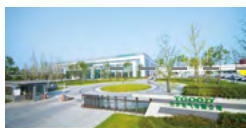
Sichuan Chengdu Manufacturing Factory
