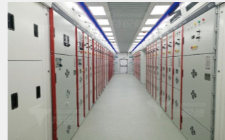
Interior Design: > Rock wool board walls + aluminum alloy grille ceiling
