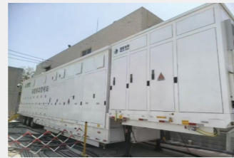
Assembled-Frame Prefabricated Substation
