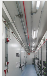
Interior Design: > Rock wool board walls and ceiling + exposed pipelines
