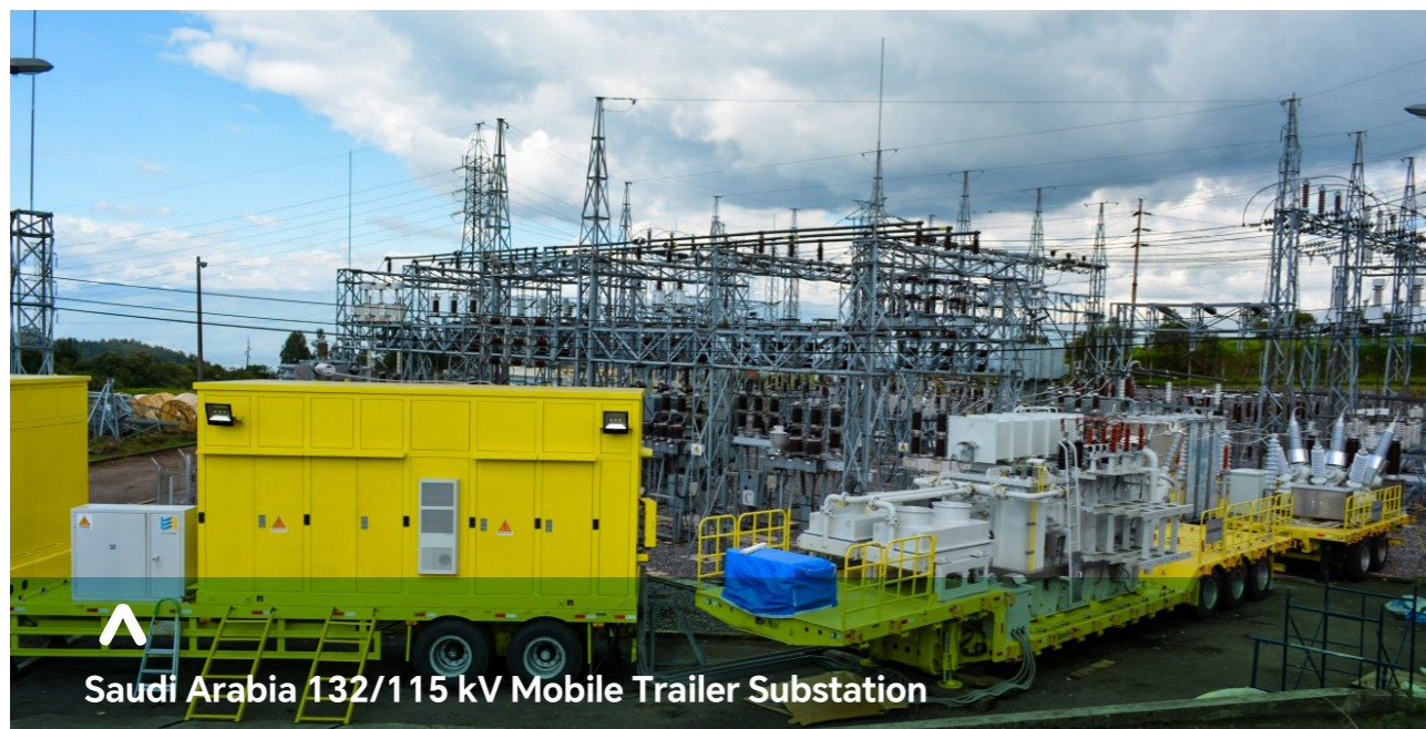
^ Saudi Arabia 132/115 kV Mobile Trailer Substation
