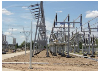
Double busbar arrangement
