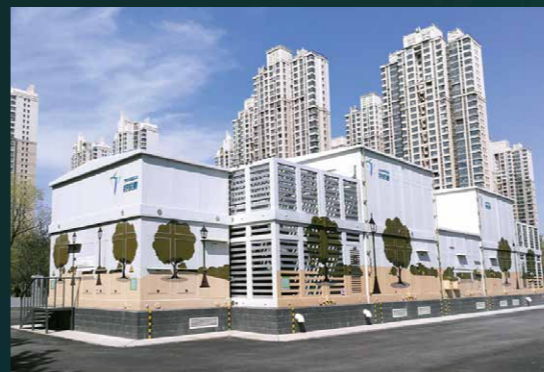
New construction of substation
