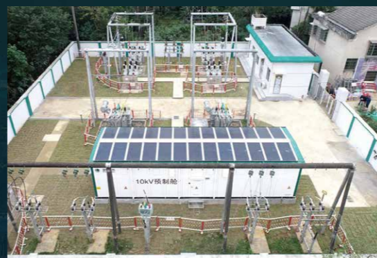
Substation technical renovation
