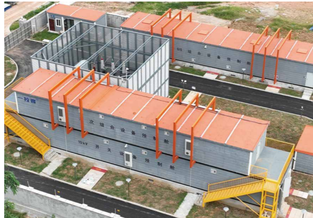
✔ Data Center Industry
