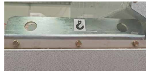
View of Switchgear Lifting
