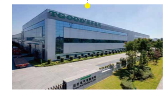
Sichuan Chengdu Manufacturing Factory
